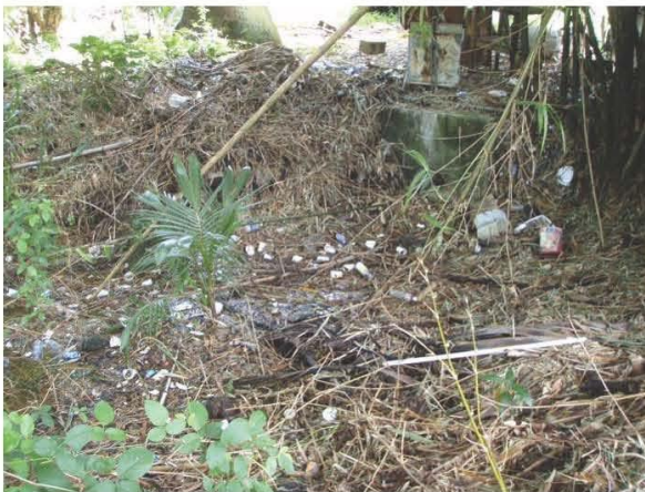
Figure D-21. Water collects in small side parking lot. Install trench drain to convey water to existing swale (top photo). May need to excavate swale to appropriate depth for trench drain invert to achieve positive drainage. Enhance swale with vegetation (middle). Trash in wetland area (bottom).
