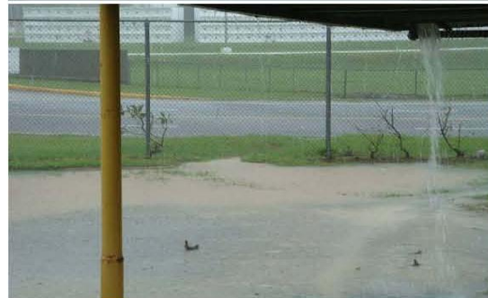
Figure B-5. Sediment in runoff is conveyed over the courtyard, into a channel then trench, and continues out across the parking lot. Runoff leaves the site and enters the street conveyance system (ditch), carrying sediment to the bay.
