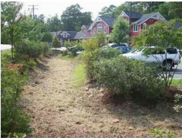
Figure D-14. Example of a surface sand filter treating parking lot runoff.
