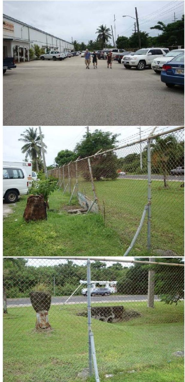
Figure D-1. Runoff from portion of rooftop and front parking drain to grassed area, then through culvert under Marine Corps Dr.
