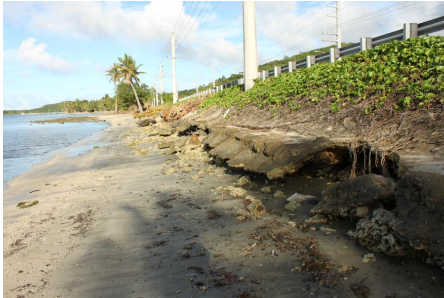
Figure 36. Eroding shoreline along Piti. Concrete was poured over limestone to stabilize the shoreline; structures are eroding and may affect the road soon.
