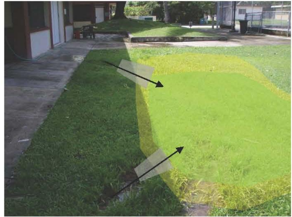
Figure D-19. Rooftop downspout through curb and onto parking lot. Washwater drains to parking lot, which drains to river (top). Proposed rain garden location in rear where roof leaders open into grassed area (lower).
