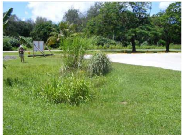
Figure D-4. Example of a rain garden treating parking lot runoff in Saipan.
