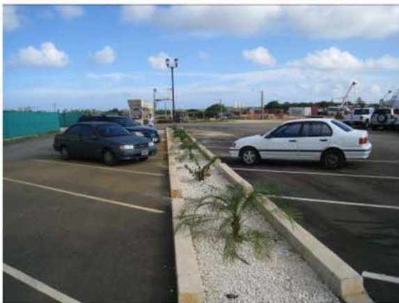
Figure D-3. Example of a parking lot bioretention area in Guam.
