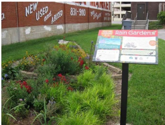
Figure D-23. Example of a small rain garden collecting rooftop runoff and accompanying signage explaining the benefits of this type of on-site stormwater management.
