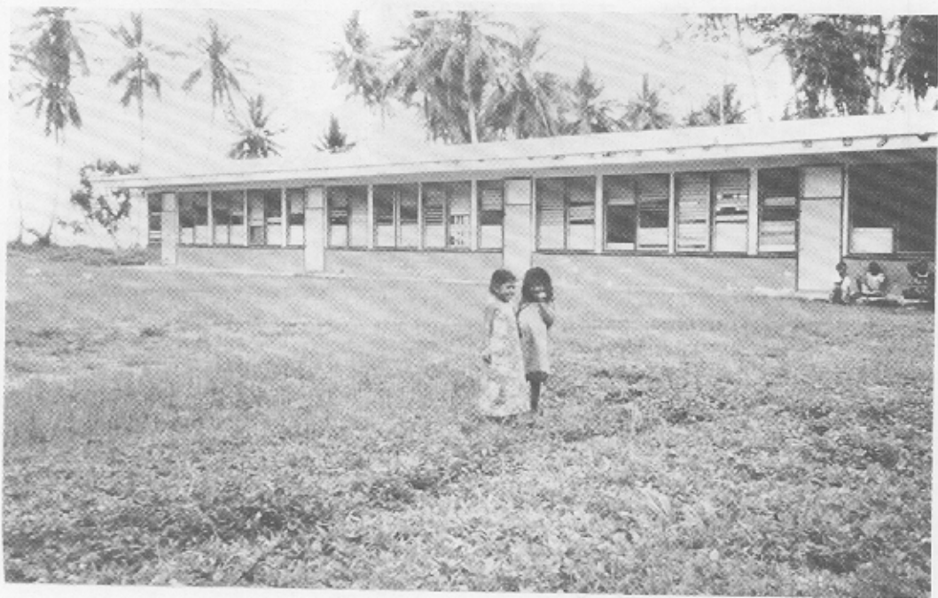
Figure 11. Typical site for "WERI WELL" installation.
