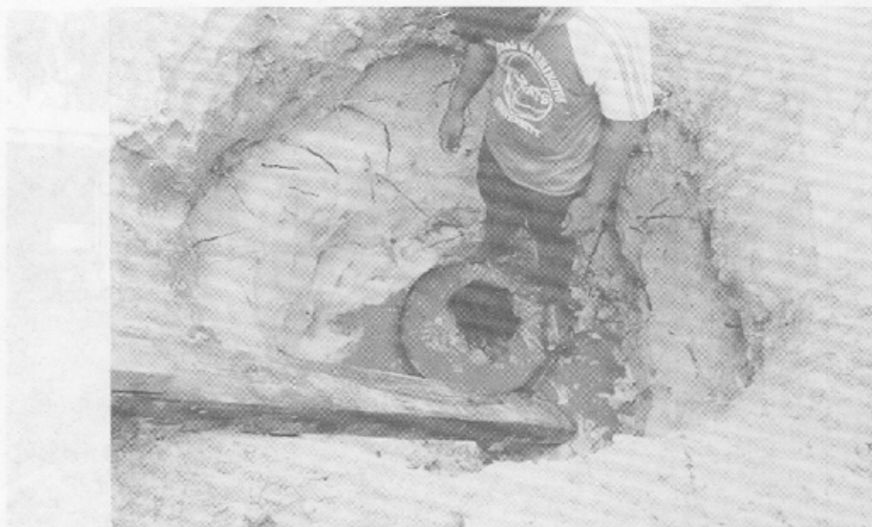
Figure 9. Digging below the water table from within a 55 gallon drum.
