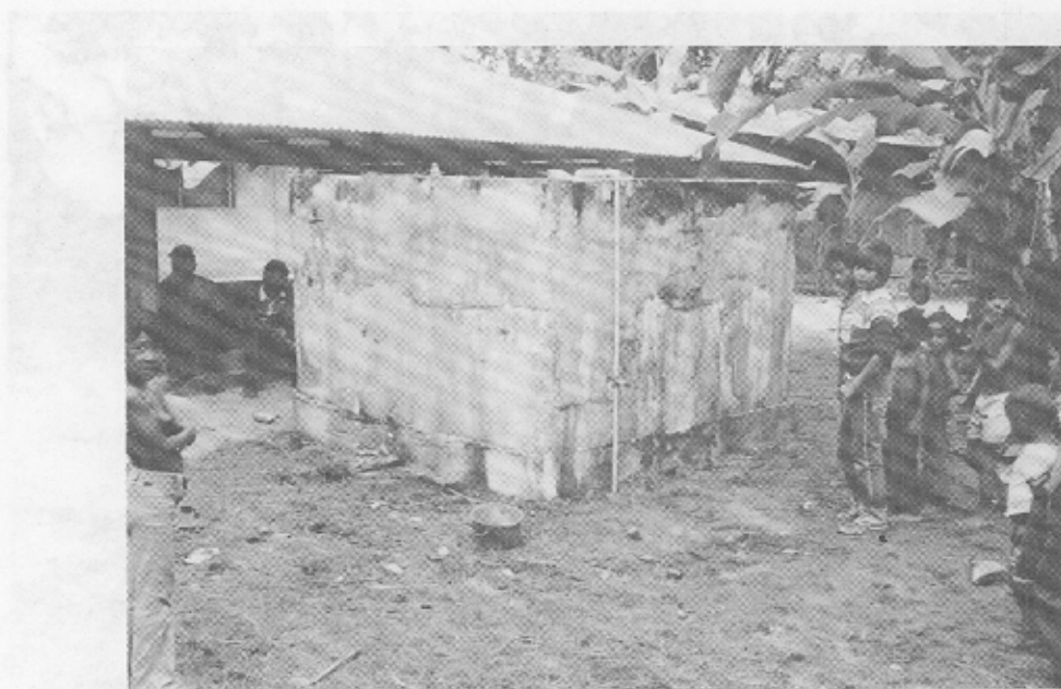
Figure 10. Typical piping arrangement and faucet location at storage tank.
