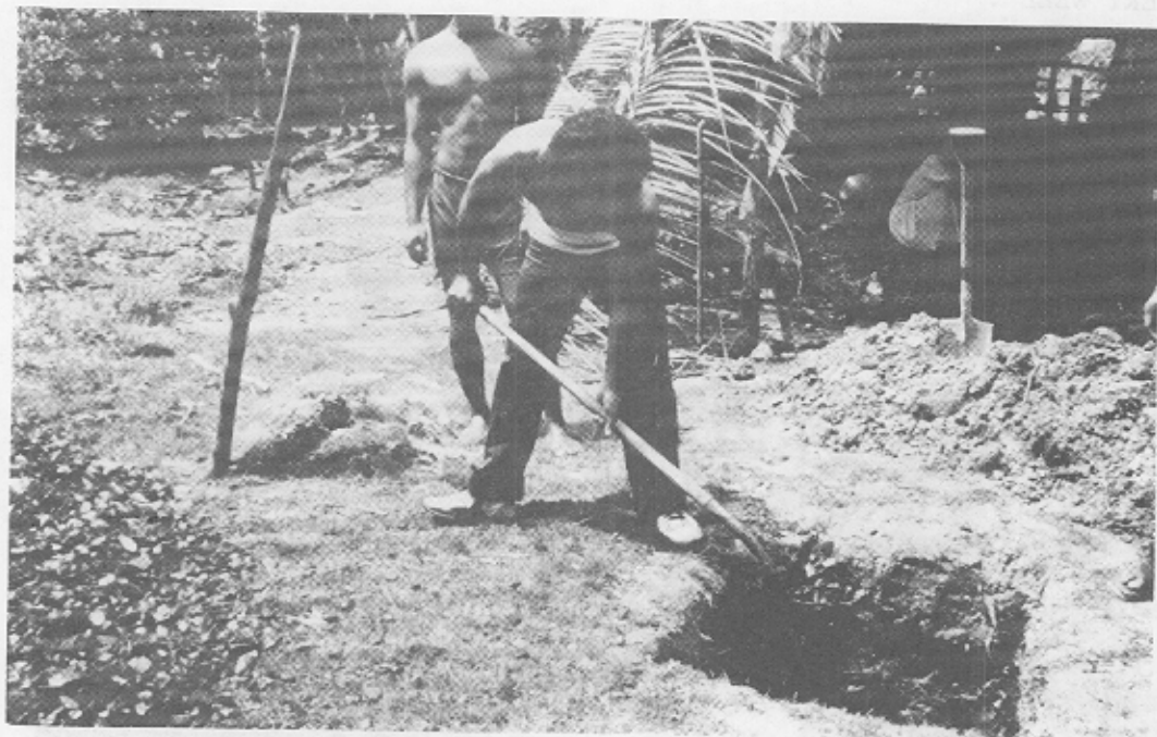
Figure 15. Backfilling with aggregate, step 1. Place about 6 inches of aggregate in the bottom of the well.
