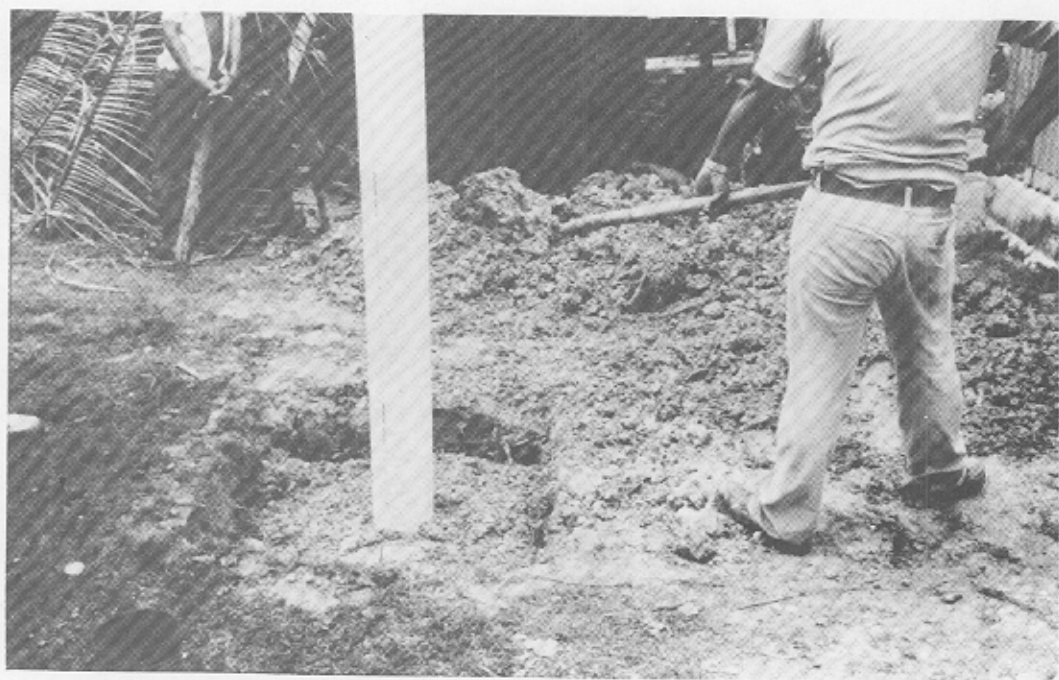
Figure 19. Backfilling with sand. Backfill the remaining portion of the well with sand originally dug from the well. Tamp it thoroughly every 6 inches.
