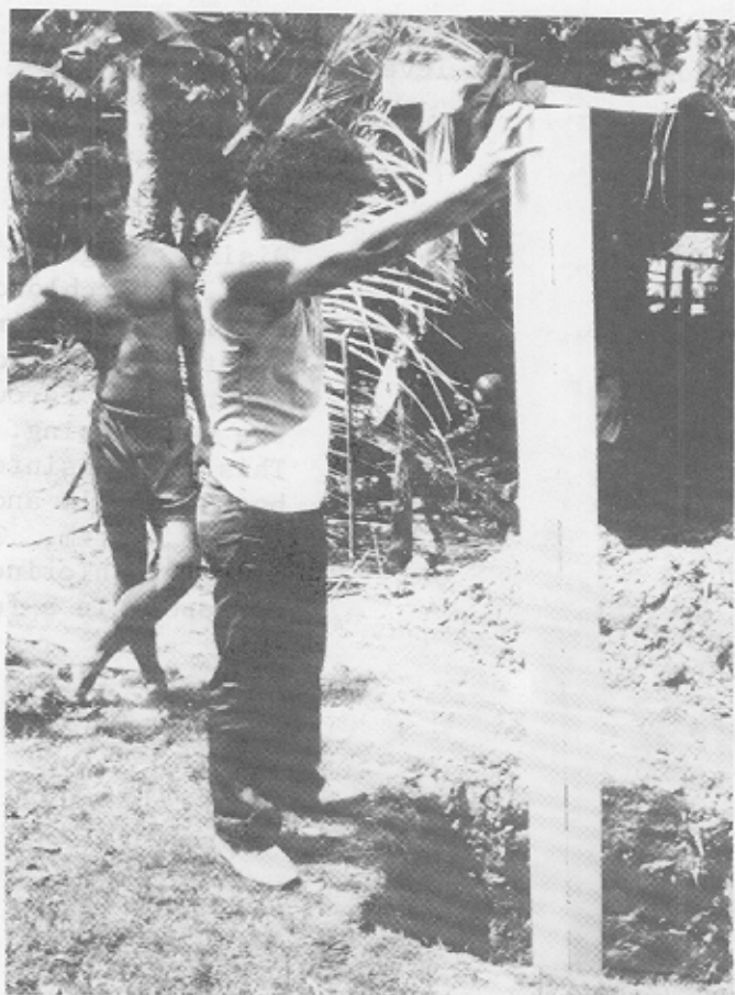
Figure 15. Backfilling with aggregate, step 1. Place about 6 inches of aggregate in the bottom of the well.
