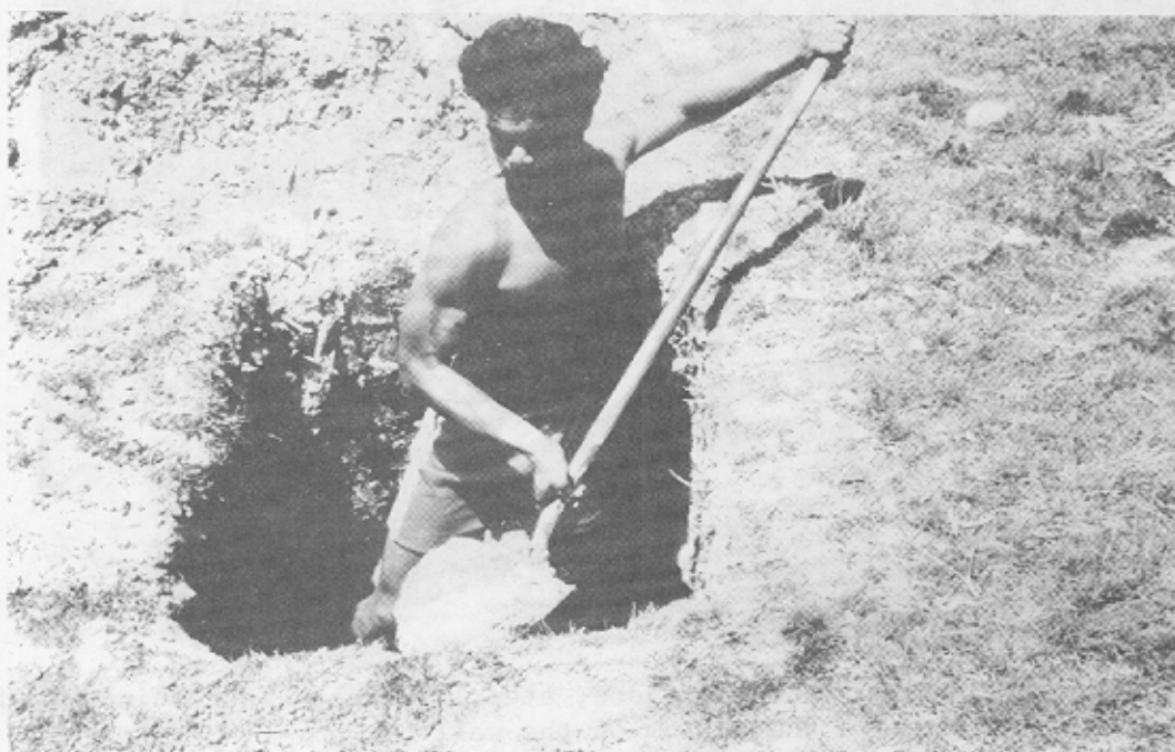
Figure 13. Digging the hole. The hole should be 3 feet by 3 feet and at least 3 feet below the low tide water level.
