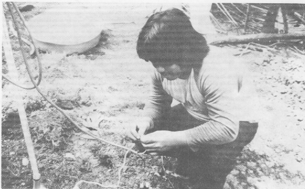
Figure 33. Connecting the wiring, step 2. Connect the white wire from the solar panel cord to the white wire from the pump cord by twisting them together. Do the same for the dark wires.
