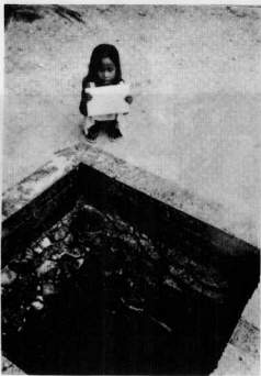
Figure 24. Well of coral blocks and concrete, Laura well #109, Majuro.
