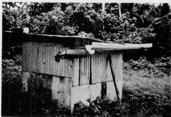
Figure 18. Concrete cistern apart from house with its own gutter, Laura, Majuro.
