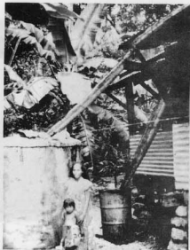
Figure 39. Concrete cistern and drum can connected to the roof by gutters, Nama Island.
