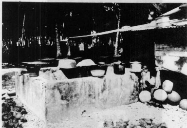
Figure 30. Old Japanese style cistern on Arno, Marshall Islands. The cistern is still used for water catchment and storage.
