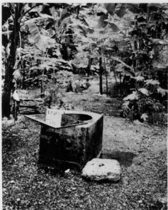
Figure 25. Well made of cement/concrete, Laura well #10, Majuro.
