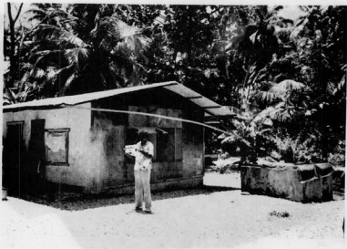
Figure 17. Gutter and cistern of concrete, close to house, Laura, Majuro.
