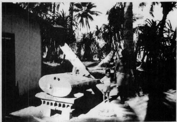
Figure 9. Rainwater catchment with an incipient gutter and semi-permanent container, Laura, Majuro.
