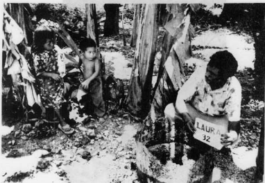
Figure 29. Well made of a drum can, Laura well #32. Drum cans frequently rust and need to be replaced.
