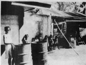
Figure 32. Attached gutter with semipermanent container, Nama Island.
