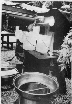
Figure 12. Attached gutter with portable containers, Laura, Majuro.
