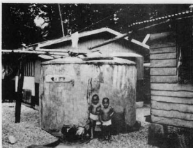
Figure 40. Gutter and concrete cistern, Nama Island.
