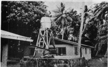
Figure 20. Concrete cistern with a raised metal water storage container on top to facilitate distribution of water. An electrically operated pump provides power for this system, Laura, Majuro.
