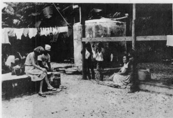
Figure 38. Concrete cistern and interview scene.
