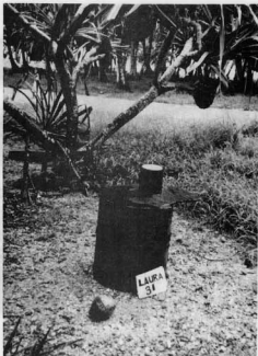
Figure 27. Well made of drum cans, Laura well #31, Majuro.
