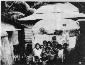
Figure 36. Concrete Cistern, Nama Island.
