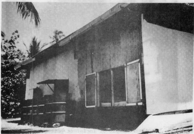
Figure 13. Attached gutter with semipermanent container, Laura, Majuro.
