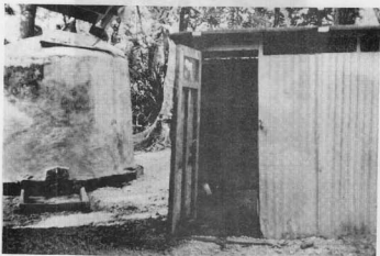
Figure 41. Toilet facility and concrete cistern, Nama Island.
