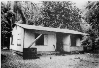
Figure 11. Another example of incipient gutter with semipermanent containers, Laura, Majuro.
