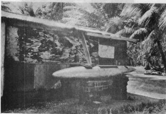
Figure 14. Attached gutter with semipermanent container, Laura, Majuro.
