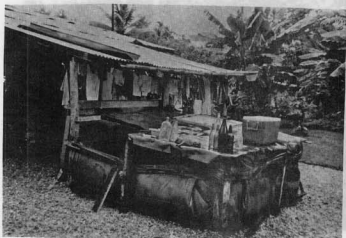
Figure 16. Gutter and cistern made of rubber, Laura, Majuro.
