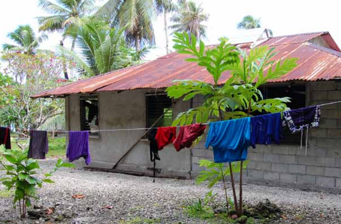
Fig 16 A typical concrete house with a tin roof.
