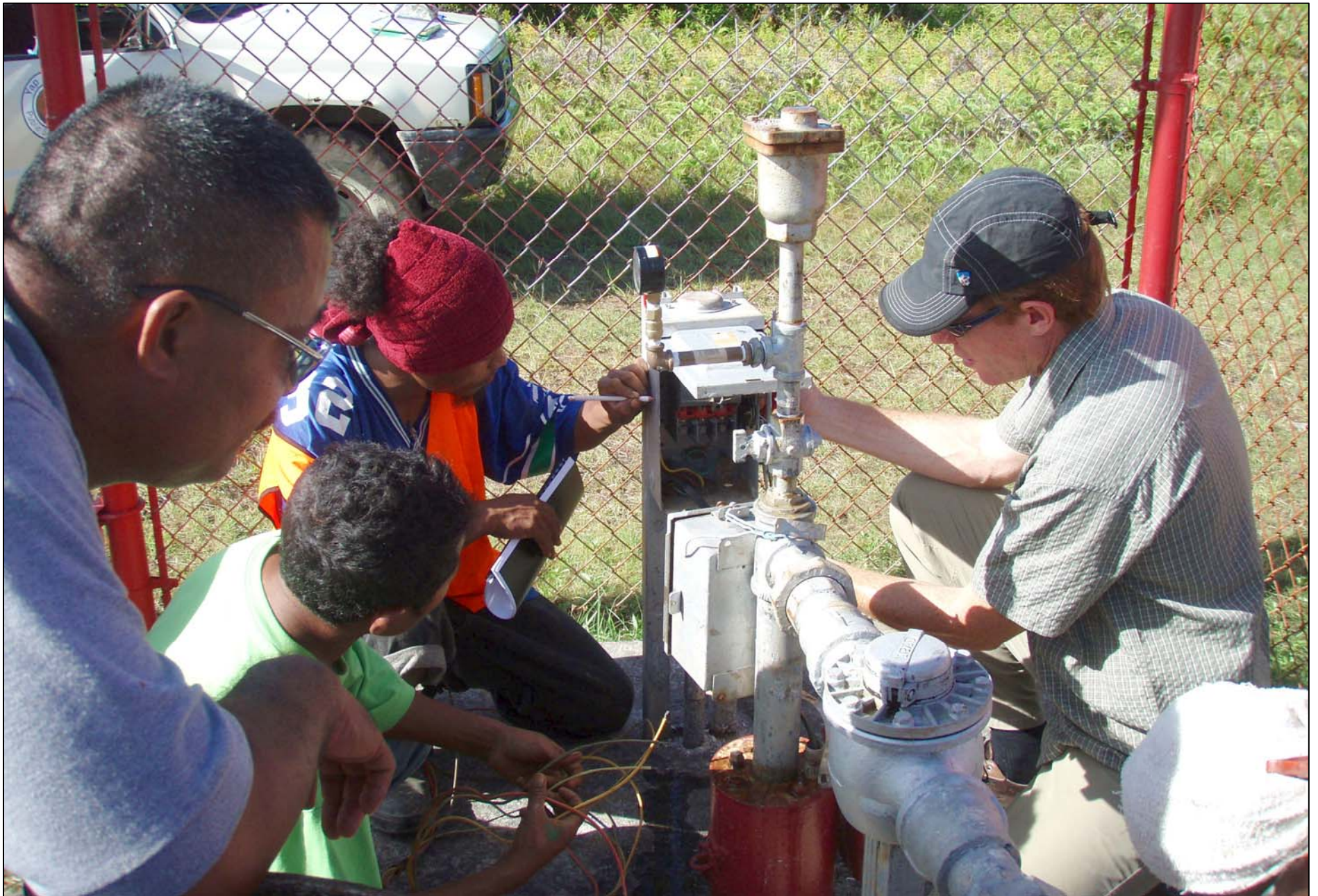
WERI conducts a Water System Operation and Training Workshop for water resources professionals in Yap State, December 2007.
